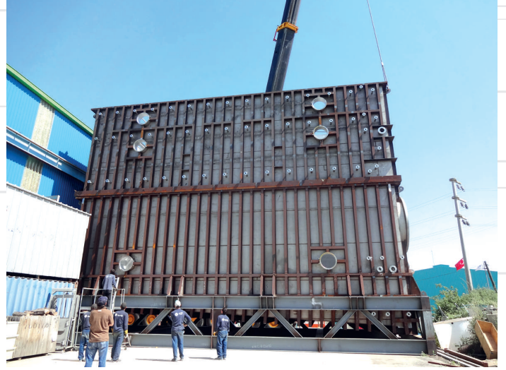
Rectangular Gas Scrubber during pre-assembly
