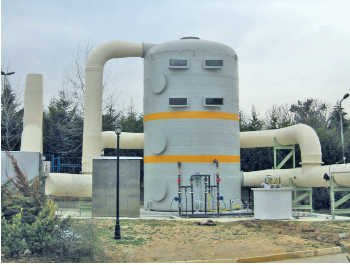
Bio-Scrubber for odour control system
