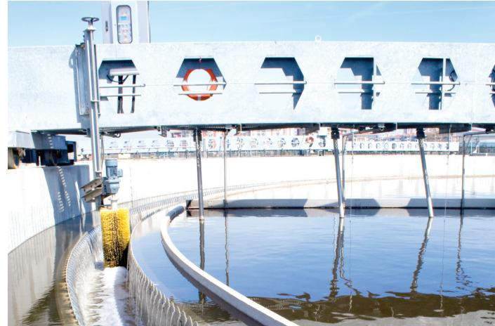
*Detail from effluent channel cleaning brush*
