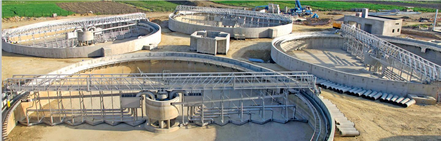
*Suction Scraper with Aluminium Truss Bridge*
