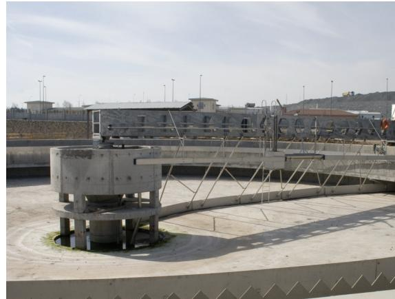
*Peripheral Driven Scraper Bridge with surface skimmer*
