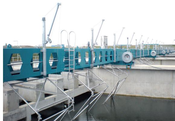
*Travelling Scraper Bridges with liftable bottom blade scrapers*
