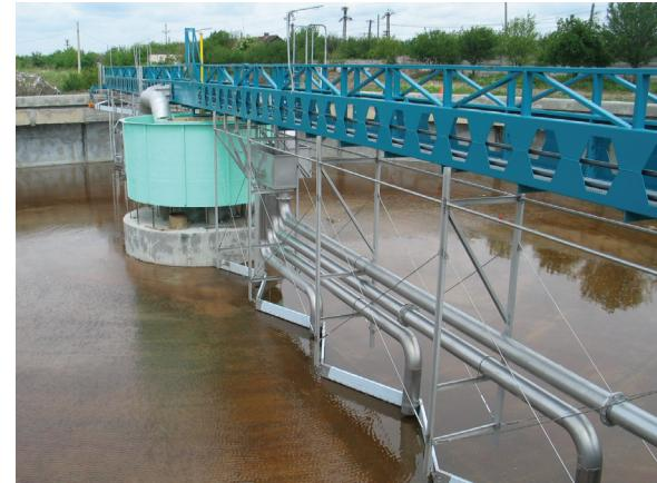
*Suction Scraper spanning the full diameter of the tank*
