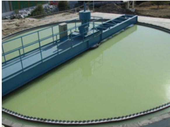
*Thickener with automatic lifting unit against overload*
