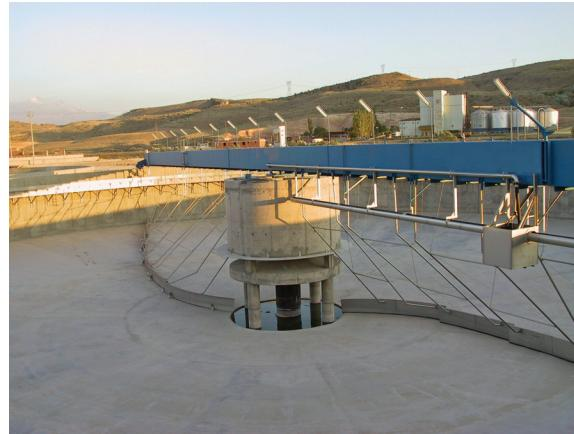
*Rotating Full Bridge with blade scrapers*
