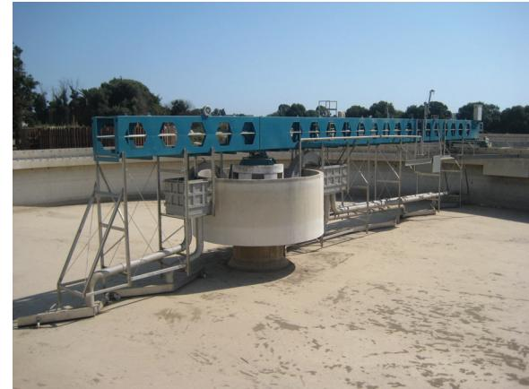
*Rotating Bridge with suction type sludge removal*
