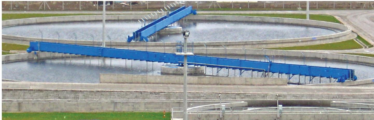
*Rotating Full Wall Scraper Bridges spanning Ø 60m diameter Sedimentation Tank*
