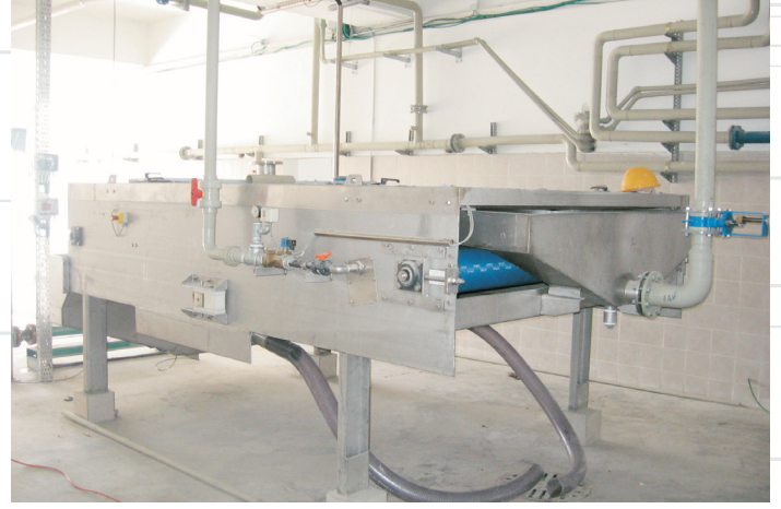
Gravity Belt Thickener during installation
