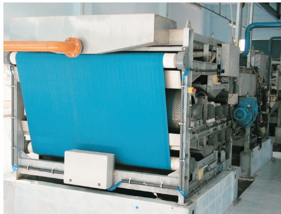
Belt Filter Presses during installation
